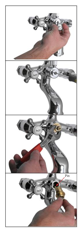
Before replacing diverter be sure the water is turned off. 1. • Remove cap from diverter mechanism. • Unscrew diverter handle. 2. • Using a wrench, loosen diverter mechanism from 3. faucet body. • Remove diverter mechanism from faucet body.
